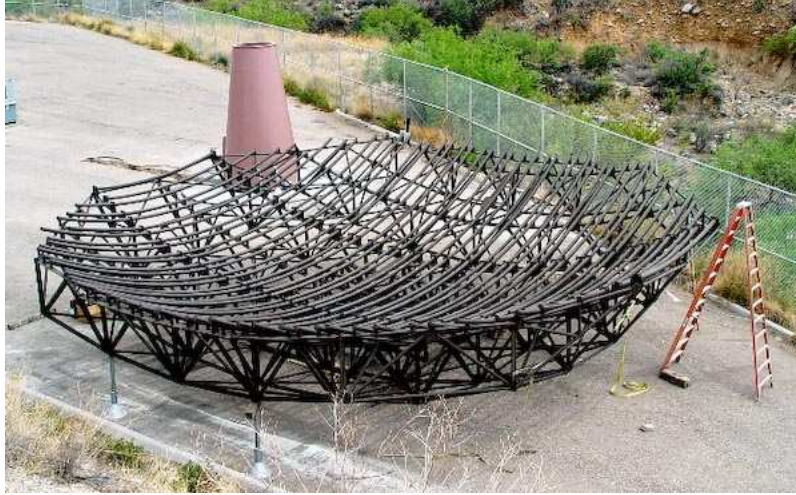
Figure 3–9: Photograph of a VERITAS optical-support-structure during the telescope construction phase.
