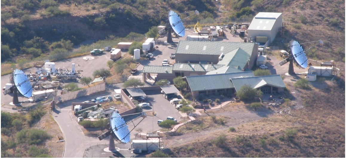
Figure 6.1: The VERITAS array at the Fred Lawrence Whipple Observatory. The array configuration seen here is the new (post-Summer, 2009) configuration which leads to relatively uniform separation distances (roughly 100 m) between the telescopes.
