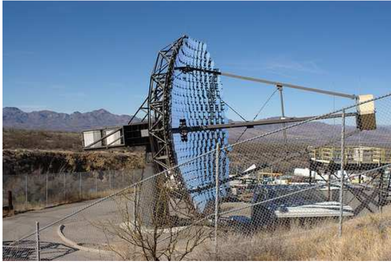
Figure 2.2: A VERITAS telescope consisting of a 12 m mirror dish mounted on a welded steel optical support structure. The camera box kept across the reflector with quadrupole arms, balanced with a counterweight at the back can be seen.
