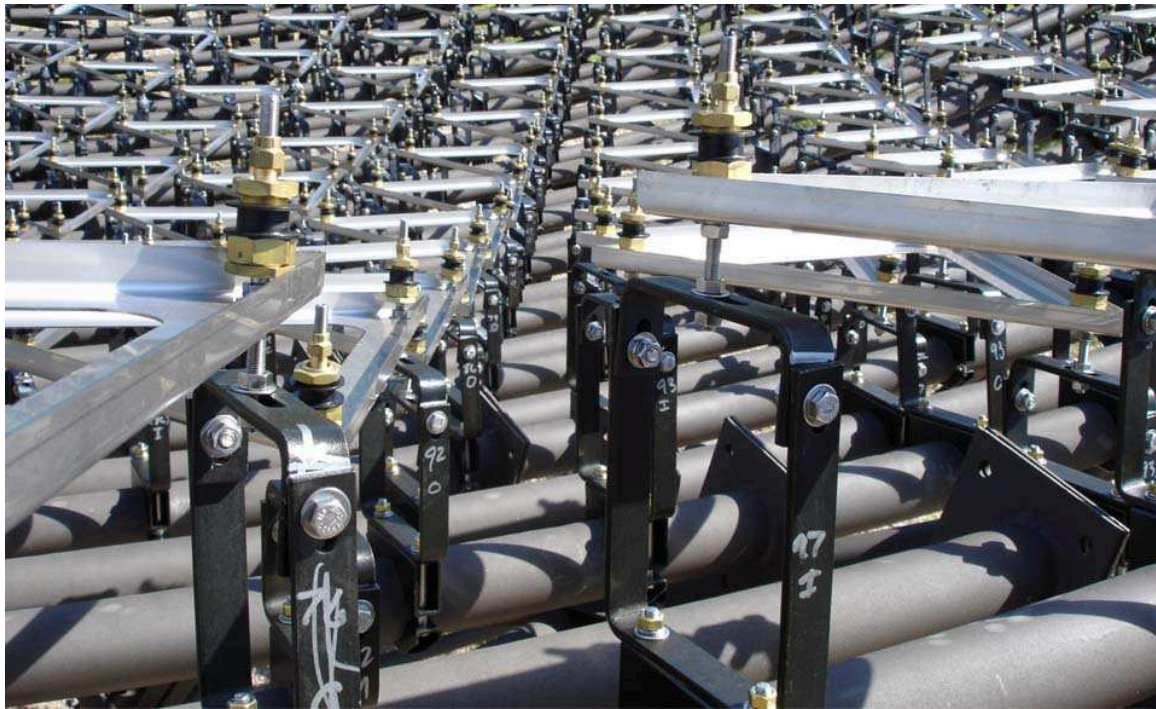
Figure 5.4: Photograph of mirror mounts. The metal triangles keep the supporting threaded rods of a mirror facet at the desired distance and parallel to each other.
