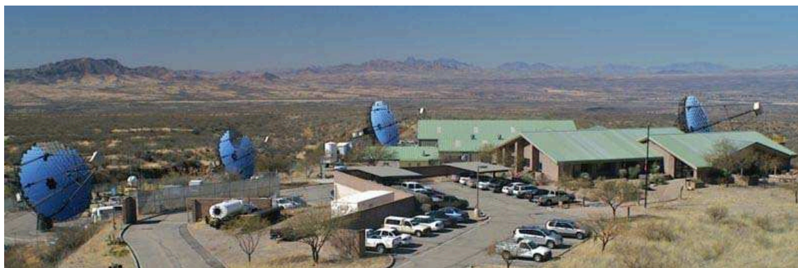
Figure 5.1: Photograph of the completed VERITAS array, located at the base camp of the Fred Lawrence Whipple Observatory. Joining the location of the telescopes with lines forms a four-sided shape with sides of lengths 85 m, 35 m, 85 m and 109 m [141].
