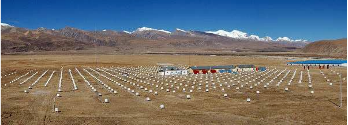
Figure 4.7: The Tibet AS-gamma Experiment. Detectors of particles are deployed over a large field at mountain altitude (4300 m above sea level). Figure taken from http://www.icrr.u-tokyo.ac.jp/em/index.html .
