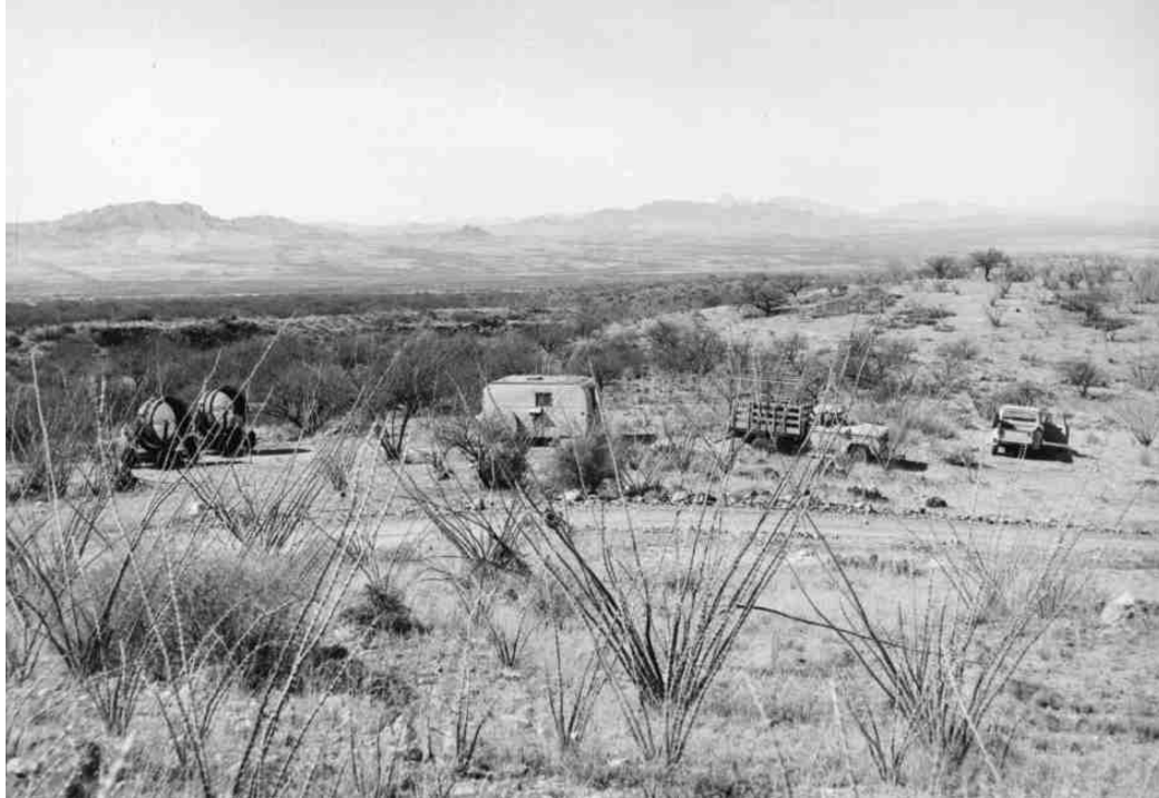
Figure 1.5.: The very first TeV gamma-ray observatory in the United States was derived from World War II searchlight reflectors, which are visible in the picture on the left. The telescopes were manually operated by eye and were located at a dark site in Arizona south of Tucson, during the winter of 1967-1968. Just by chance, they were located exactly at the same place where the VERITAS telescope array is currently located [7].
